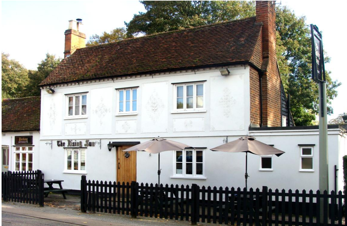
Picture 13. The Rising Sun PH. Although compromised to some degree by later extensions its general mass and chimney features are important in the street scene that should be retained.
